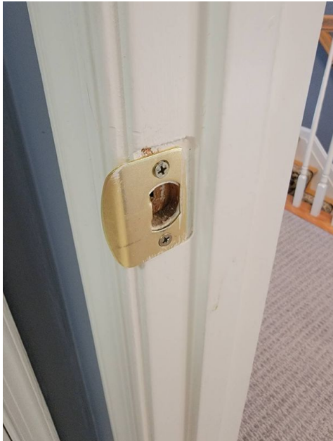
Strike Plate needs Adjustment
