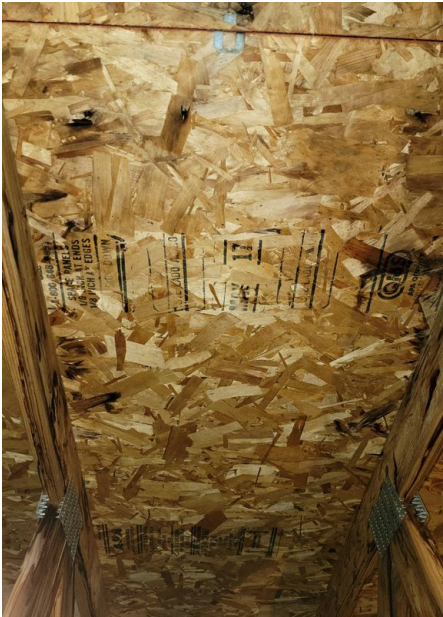
OSB Oriented Strand Board Sheathing
