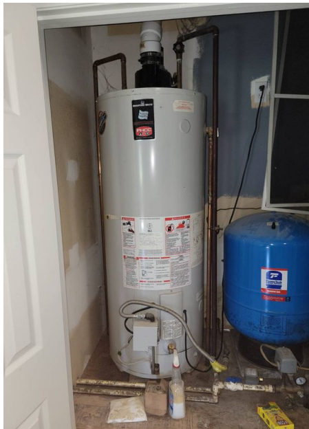
High Efficiency Water Heater (Propane)
