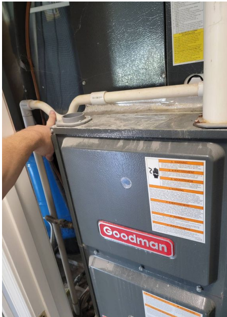
Condensate Drain Line (Goes into Crawl Space)
