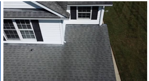
Roof in Serviceable Condition
