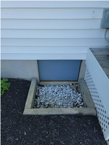
Crawl Space Access(Left Side)
