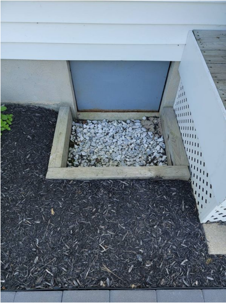
Window Well Drainage (Left Side)
