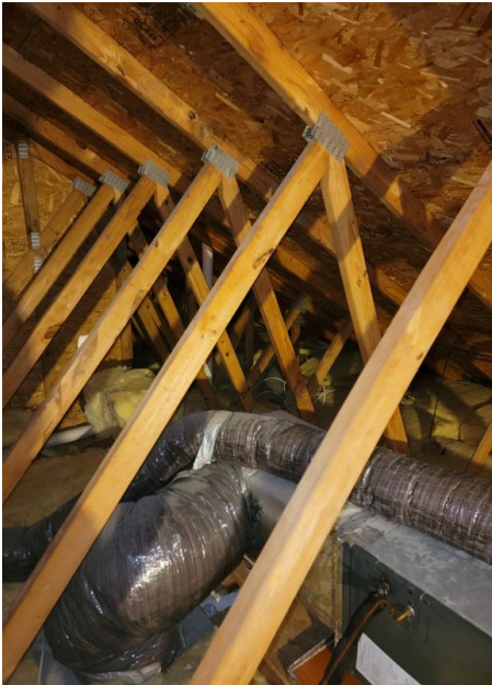
Roof Structure Engineered Trusses
