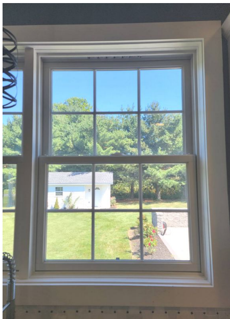
Single Hung/Thermal Insulated Wooden Windows
