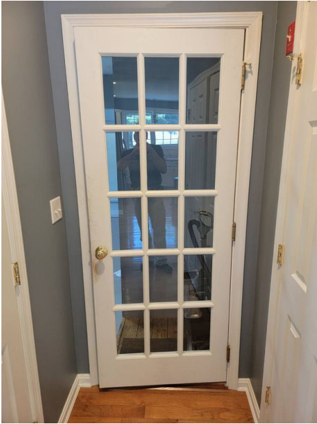
Garage Occupant Door (See Comments)
