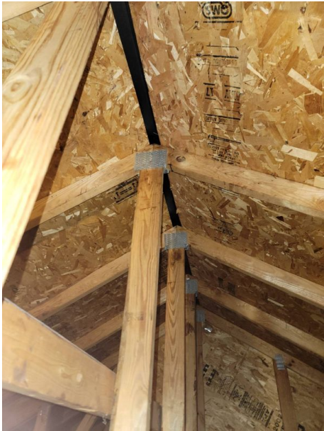
Roof Structure Engineered Trusses
