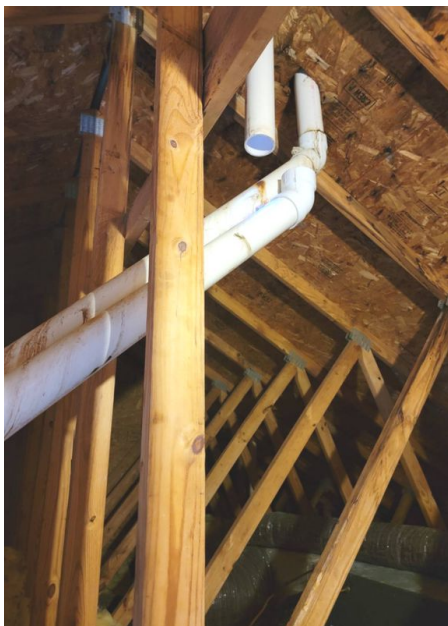
Condensate Drain Line (Goes into Crawl Space)
