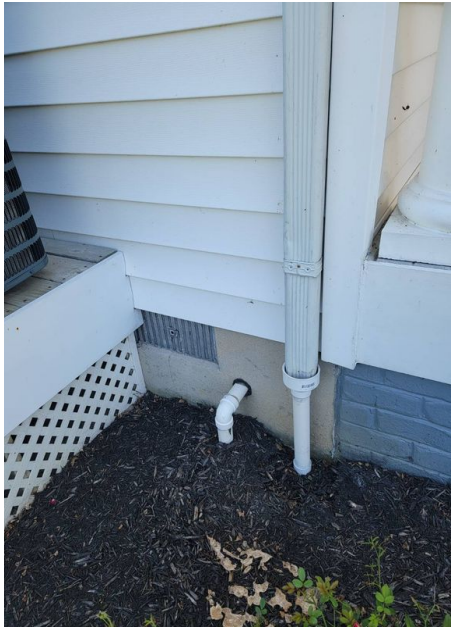
Foundation Cinder Block w/Parging
