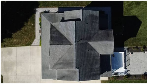
Roof in Serviceable Condition
