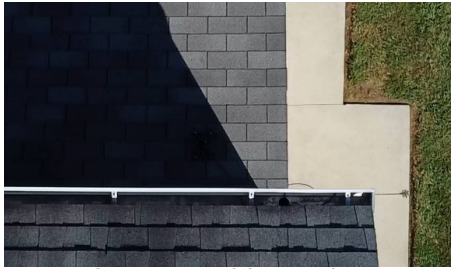
Roof in Serviceable Condition
