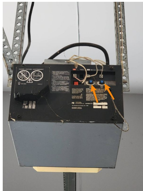
Sensitivity Adjustment for opener
