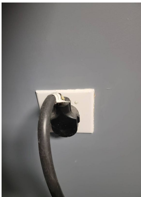
Newer 4 Prong Receptacle for Dryer
