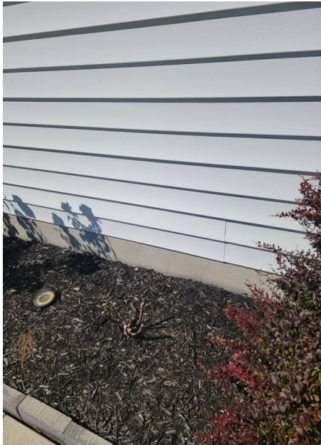
Foundation Cinder Block w/Parging
