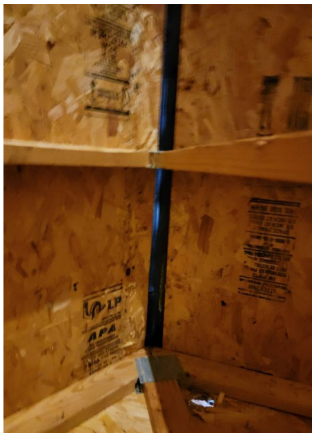
Ridge Vent from Attic
