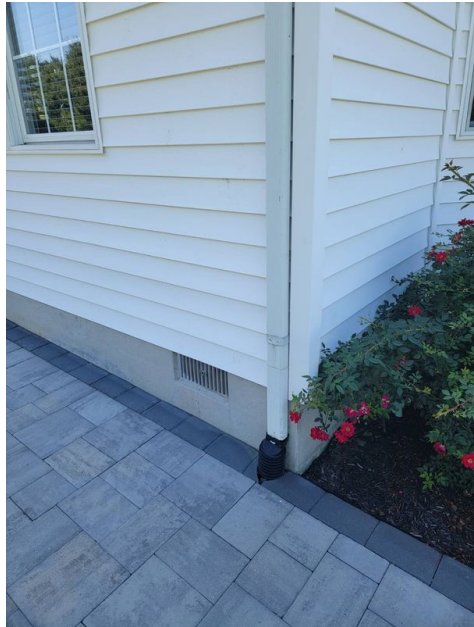
Foundation Cinder Block w/Parging
