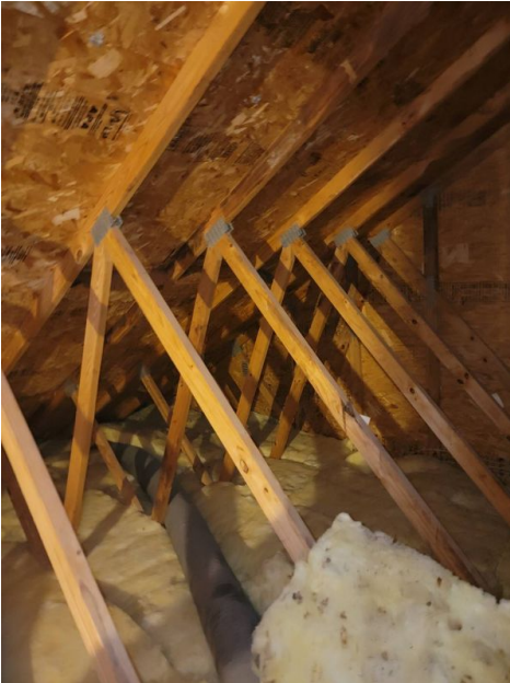
Roof Structure Engineered Trusses
