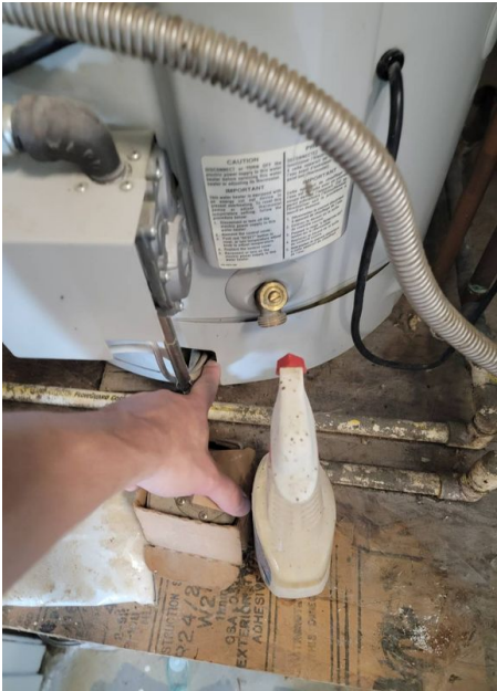
FVIR Propane Tank
