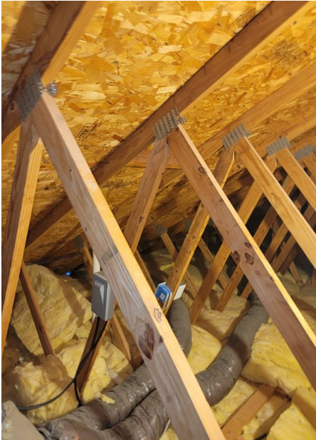
Roof Structure Engineered Trusses
