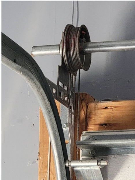
Safety Cables Good to See
