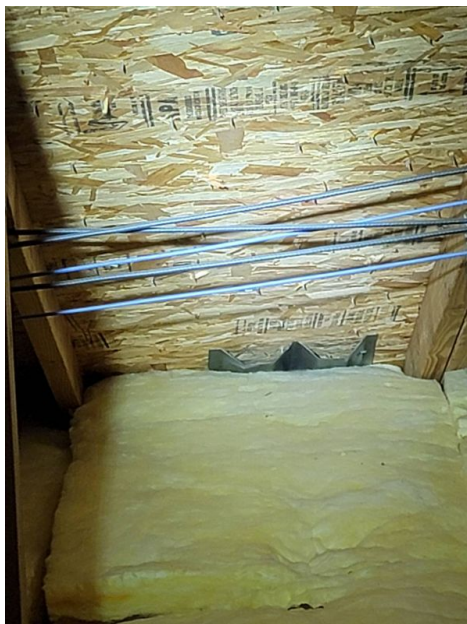
Soffit Baffles Allows for Functional Ventilation
