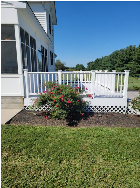
Lattice Restricts Inspection Below Deck All around Bottom
