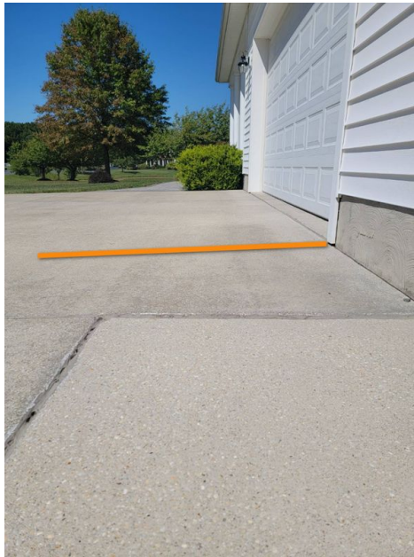
Grading(Front) Away from Foundation Acceptable
