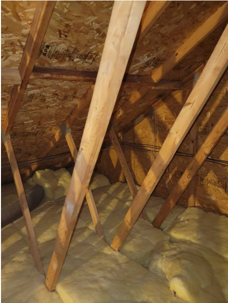
Roof Structure Engineered Trusses
