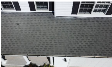
Roof in Serviceable Condition
