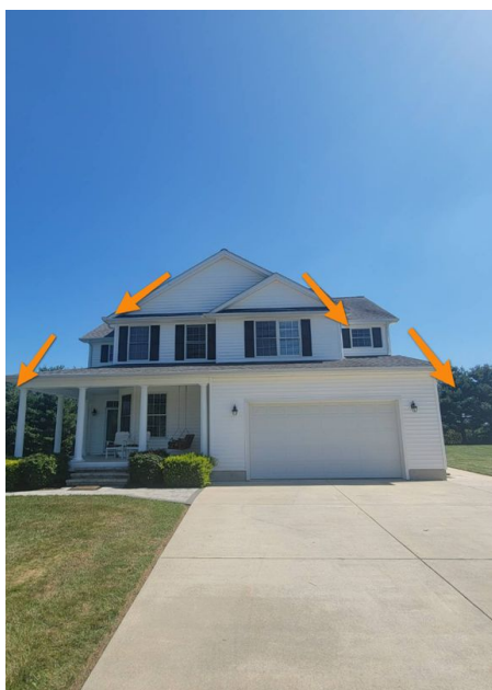
All Gutters Pitched Properly Toward Downspout
