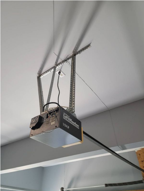
Garage Door Opener (Chain Driven)
