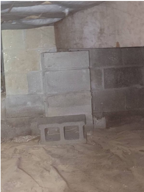
CMU Cinder Block Pier
