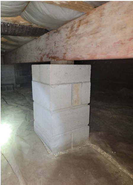
CMU Cinder Block Pier
