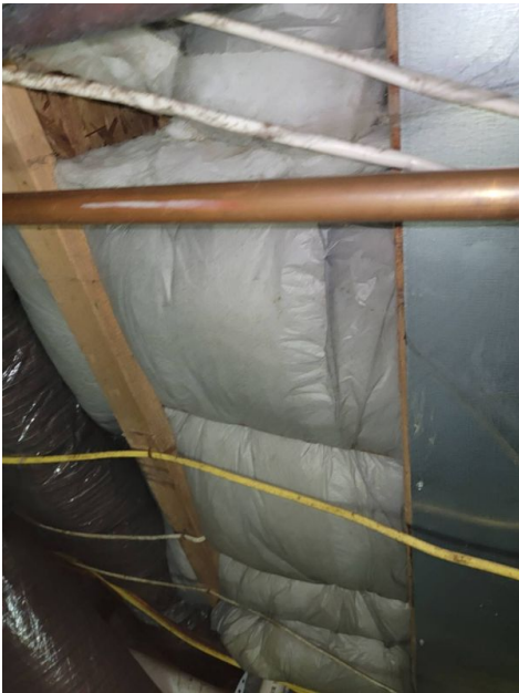
Floor structure I Joists
