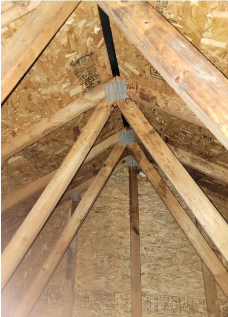
Roof Structure Engineered Trusses
