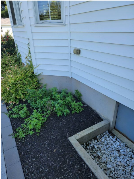
Foundation Cinder Block w/Parging
