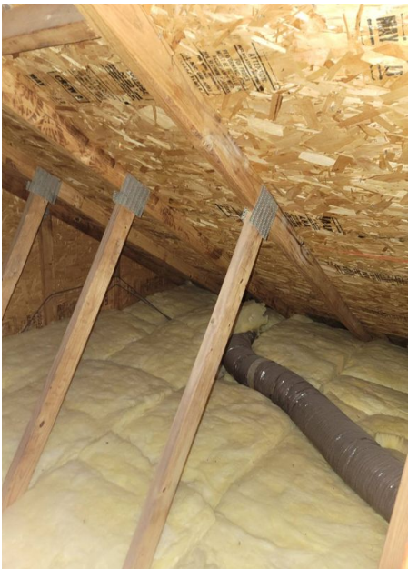
Roof Structure Engineered Trusses
