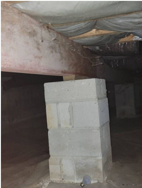
CMU Cinder Block Pier
