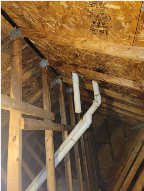
Roof Structure Engineered Trusses
