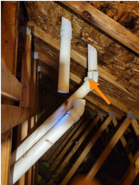
Attic Flue Pipe
