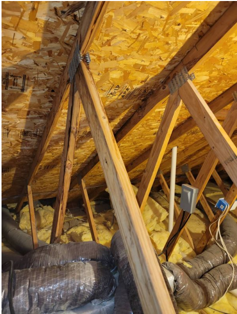
Roof Structure Engineered Trusses
