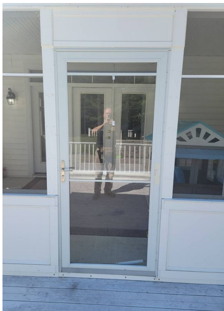
Deck Storm Door Composite/Tempered Glass
