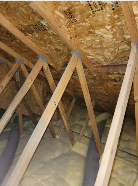
Roof Structure Engineered Trusses
