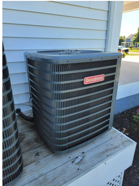
Condenser for Air Conditioner (Right Side Unit)
