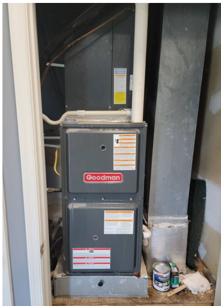
High Efficiency (Propane) Furnace
