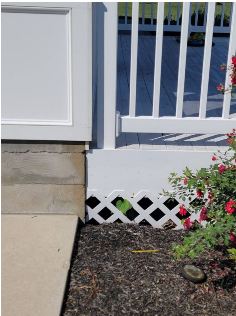
Lattice Restricts Inspection Below Deck All around Bottom
