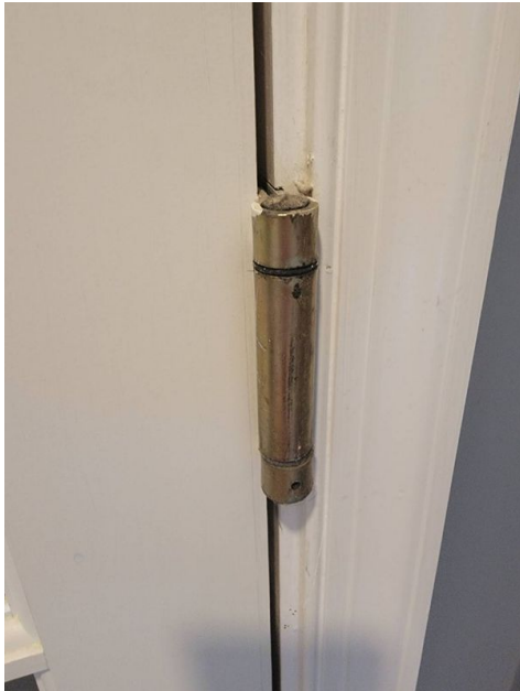
Self-Closing Hinges Exists
