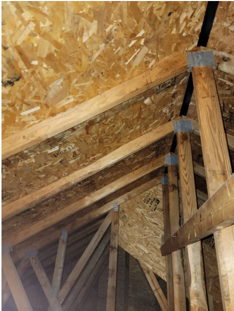
Roof Structure Engineered Trusses
