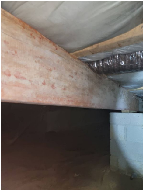
Wood Structural Beam
