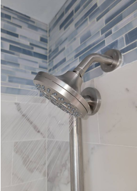
All Showerheads Passed Functional Flow Test
