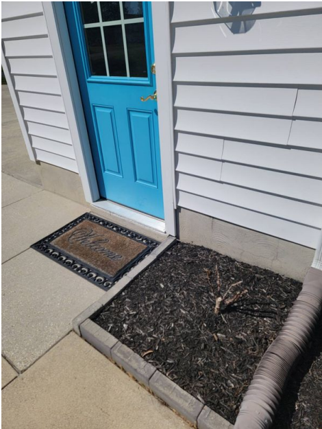
Foundation Cinder Block w/Parging
