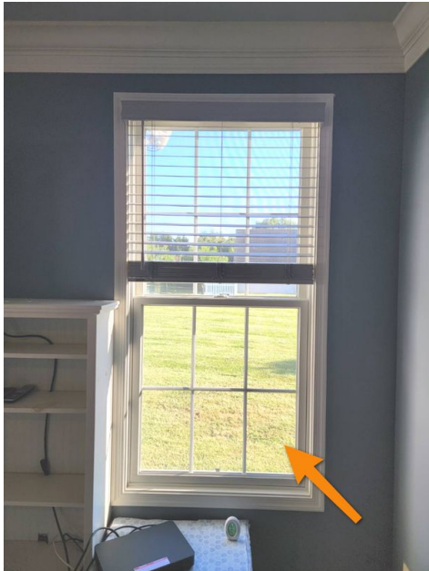
Lower Sash won't stay open(Needs Adjustment)
