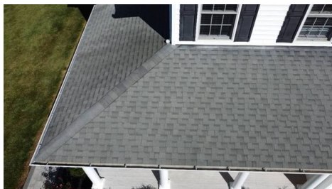
Roof in Serviceable Condition
