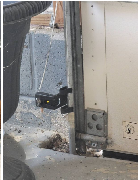
Photoelectric Auto reverse sensors (Unable to Test)
