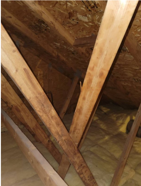
Roof Structure Engineered Trusses
