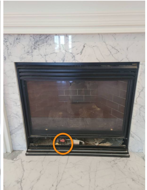
Fireplace Gas Shut-off Valve
