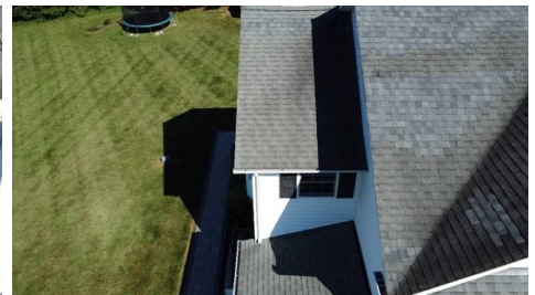
Roof in Serviceable Condition
