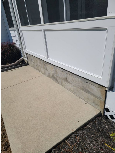
Foundation Cinder Block w/Parging
