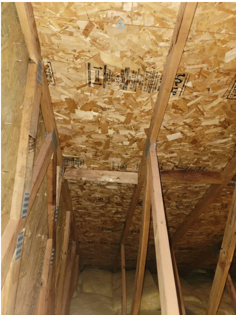
Roof Structure Engineered Trusses
