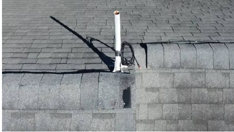
Base for TV Dish still on roof
