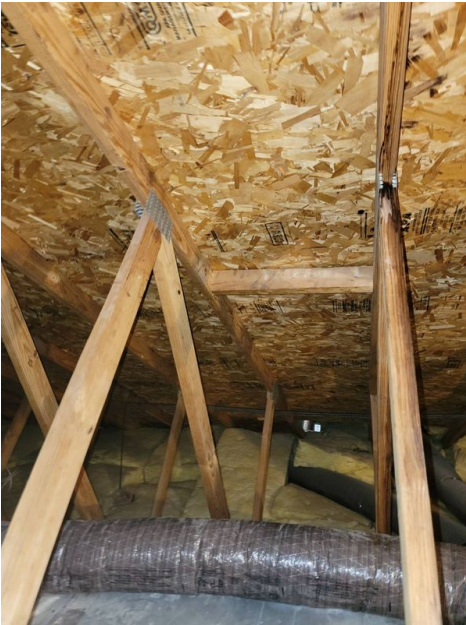
Roof Structure Engineered Trusses
