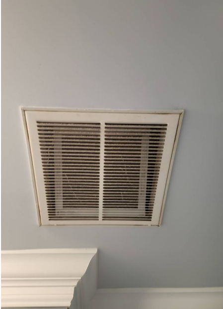
Hallway Return 14x14x1 Filter Size
