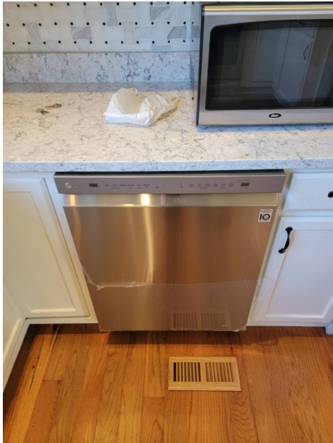
Dishwasher is Loose(Not anchored) Functional
