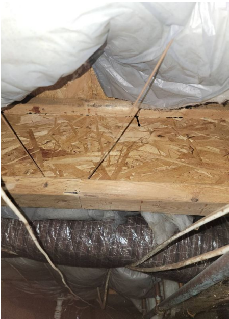
Floor structure I Joists
