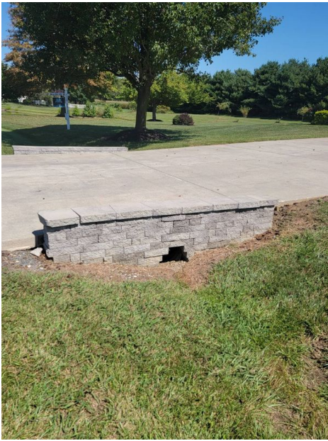
Under Driveway Drain/Swale(Maintenance)
