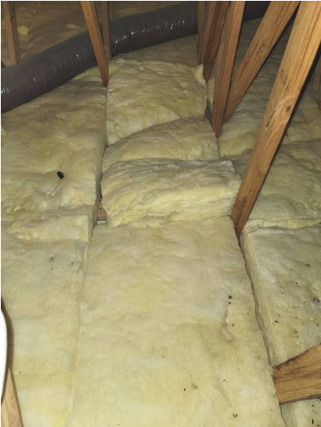
Attic Insulation Fiberglass Batts 10 inches Deep
