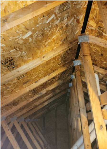
Roof Structure Engineered Trusses
