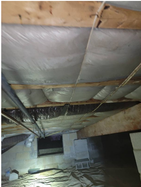
Floor structure I Joists
