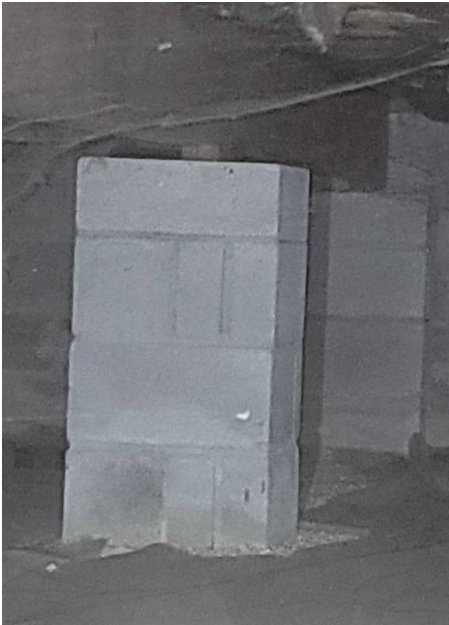
CMU Cinder Block Pier
