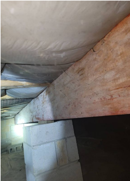
Wood Structural Beam
