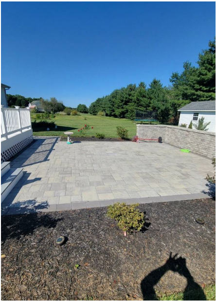
Rear Patio Concrete Pavers
