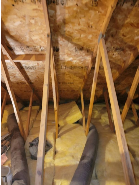
Roof Structure Engineered Trusses
